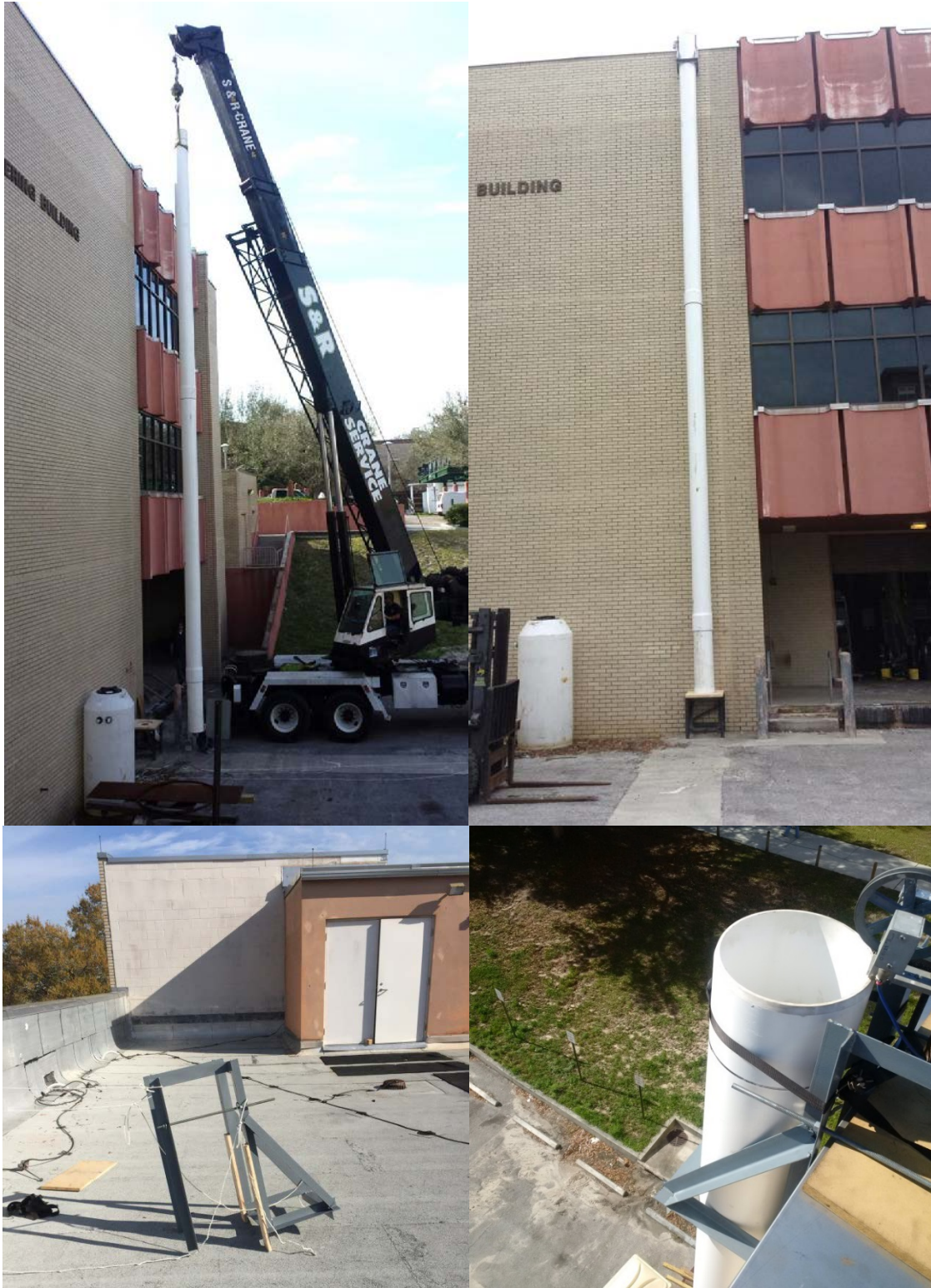
Figure 5.2. Final positioning and fastening bracket bolted to top of building.
