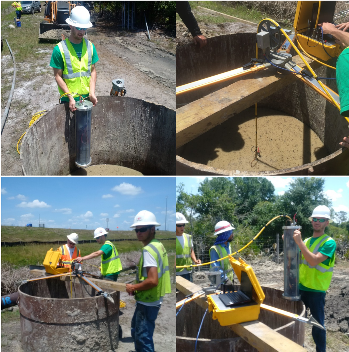
Figure 5.14. Slurry testing at I-75 Harborview Rd high mast light foundation.
