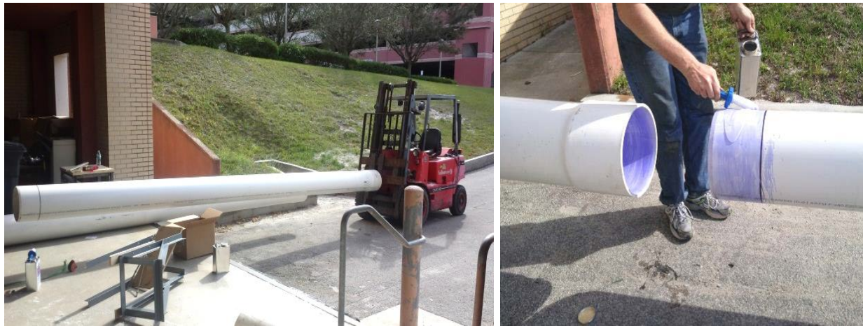
Figure 5.1 Assembly and erection of 45ft field simulation vessel
